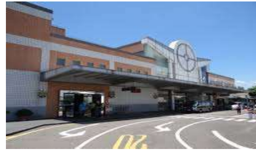
Tainan Airport Station 200RT X 2 (2016.9)
