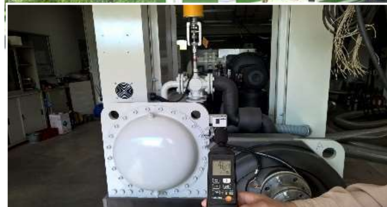
ITRI Guangfu New Bldg. 200RT (2017.1)
