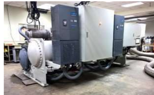
TaiPower Building 400RT (2016.2)
